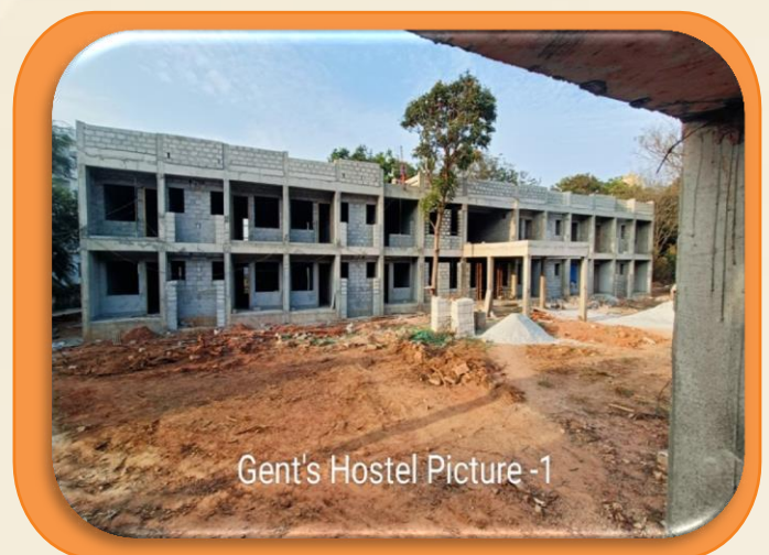
Under construction hostel at RPWTI Bengaluru.
