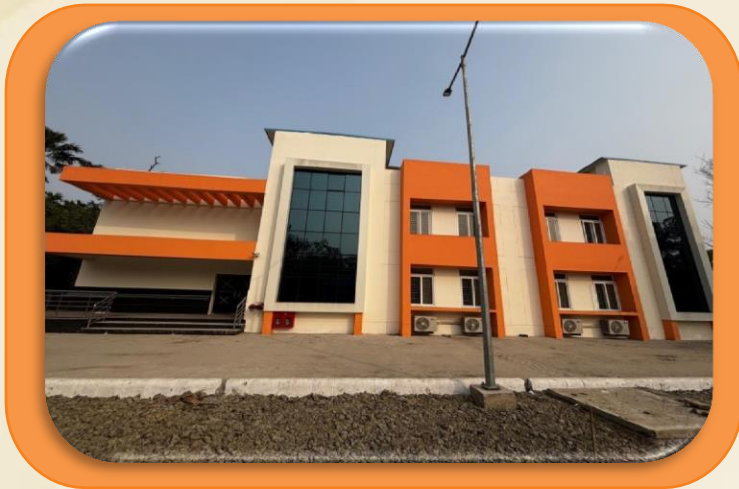
Newly constructed building at RPWTI Kolkata.
