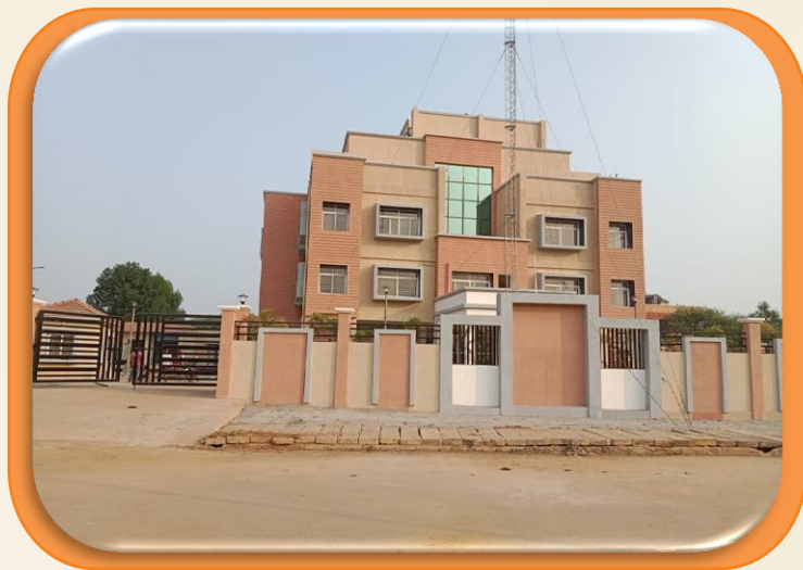
Under construction office building at ISPW Raipur.
